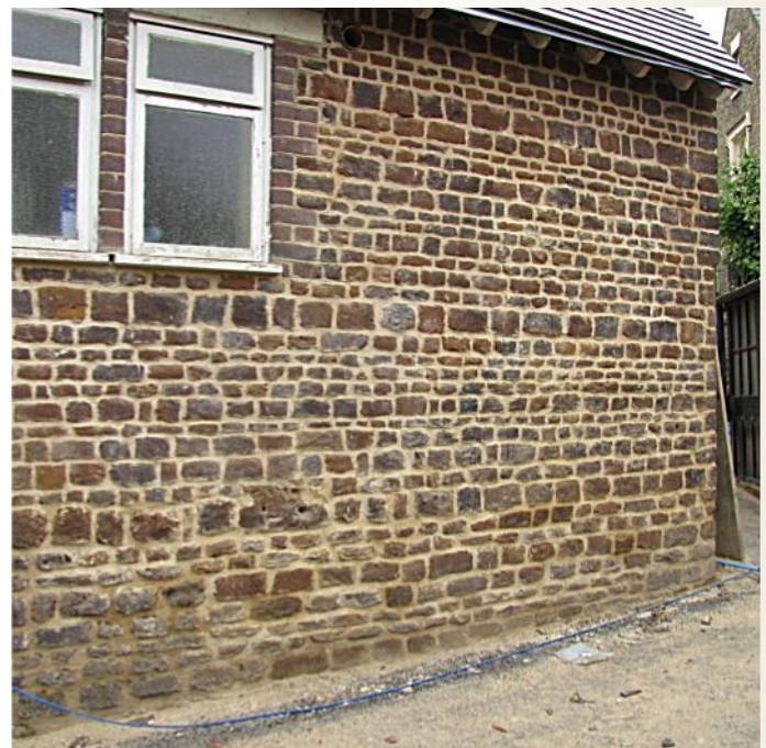
South Wall Restoration : see March N/L
